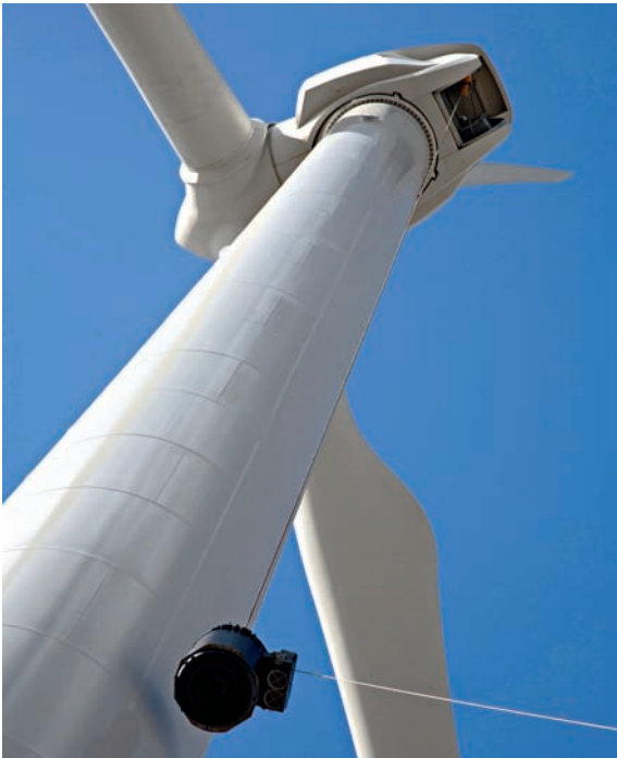
Weight lifting Removal of one of four generators in a Clipper 2.5 MW turbine via an onboard jib crane
