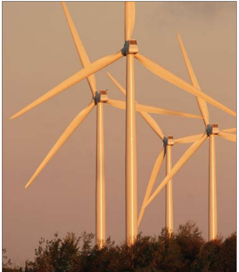
Energised by mandate: To get built, Horizon's 300 MW Maple Ridge plant needed green credit customers. They did not appear until New York state passed its RPS law
