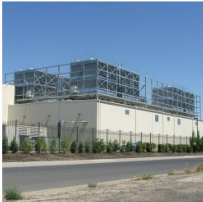
Google's data center in The Dalles, Ore.
